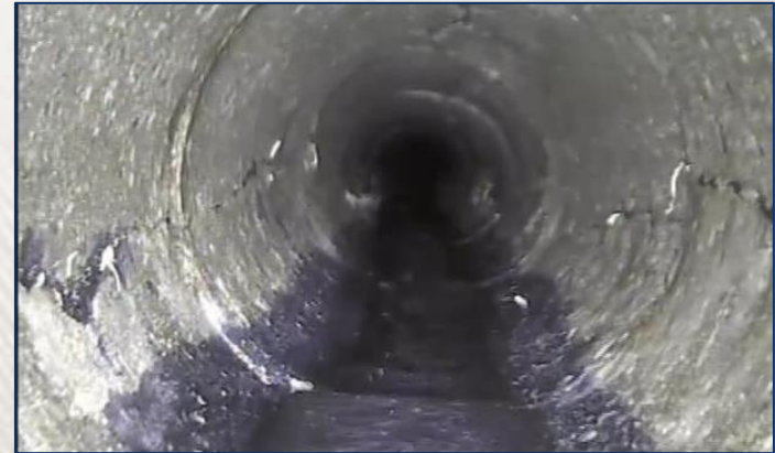
Before Trenchless Rehab
