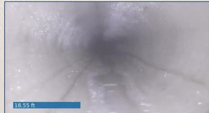
After Trenchless Rehab
